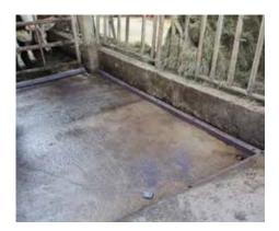
first, the border of the area is laid out with frame profiles
