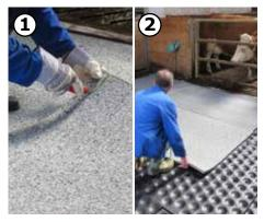
...then foam parts are placed on the and now the top covering is rolled lower mats
