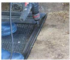
finally the covering strips are fastened on the top covering with spax screws
