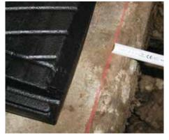
from the rear concrete edge the installation distance is marked and the mats are aligned to it
