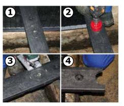
then the pockets for the pipes are marked on the profiles and cut out
