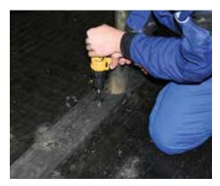
since the profiles are divided, an additional countersink must be set for fastening
