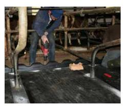
finally ergoBOARDS are installed at the front mat edges as brisket boards
