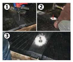
the profiles are fixed at each countersink, the screws are not yet fastened tight
