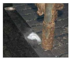
the mat edges of both outer mats are fastened afterwards with profiles
